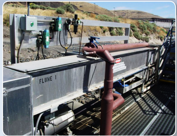
Separator Slide Gate at Lower Monumental Lock and Dam.
